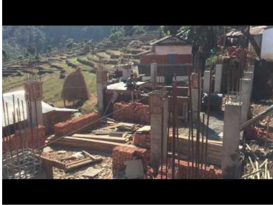
Rebuilding of the school
